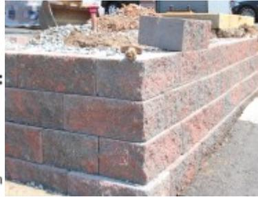
Shown is a Cambridge Sigma 6-Inch raised patio retaining wall in the full setback configuration with Cambridge Large Caps. The Sigma 6-Inch Wallstones can be set almost vertically (1.6 degree) as well as full setback (6 degrees) for additional strength. These instructions cover the following: The corner structure and the adjustment wallstone for bond as the wall is built higher on each layer and adding cap stones.
